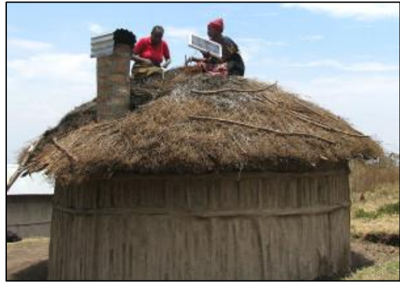
Stove and Solar fitting
